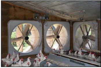
Figure 1. 55" Variable-speed tunnel fans (exterior view).
