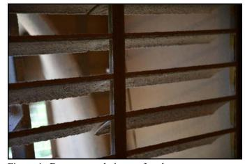
Figure 4. Dust accumulation on fan shutters.
