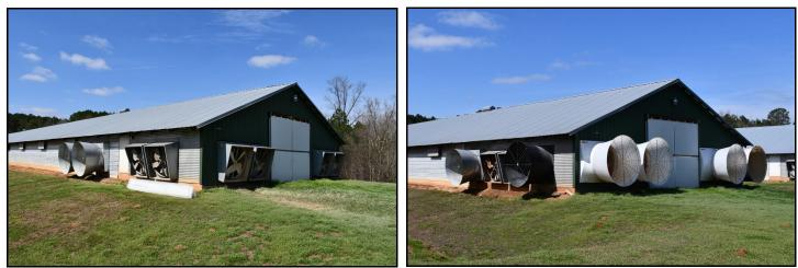
Figure 1. Tunnel-ventilated house equipped with eight 48" Figure 2. Retrofitted house where four of the 48" fans were fans and four 54" cone fans. replaced with four variable-speed 54" fans.
