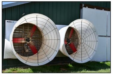
Figure 3. Variable-speed Multifan 54" Tunnel Fan.
