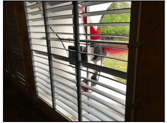
Figure 4. Interior view of fan and controller (plastic shutter was replaced with aluminum shutter after the first flock due to excessive leakage)
