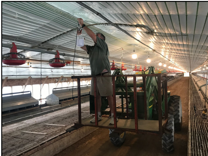
Figure 2. Installation of 40-watt LEDs
