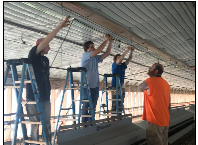
Figure 3. Installation of cord sets with sockets over nests
