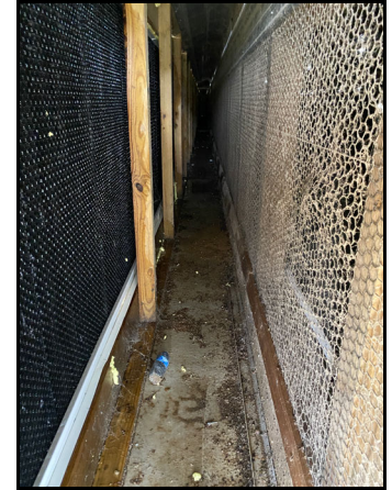
Figure 2. Wet pad room floor in house with plastic pads
