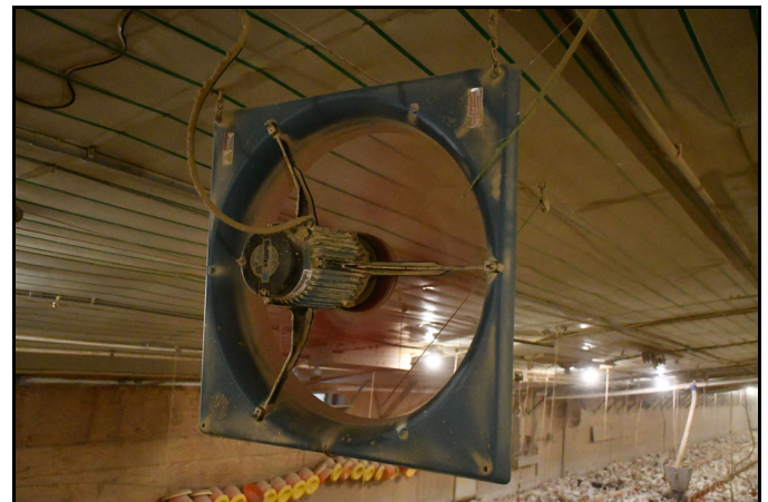
Figure 2. Circulation fan positioned at the ceiling and held so that it blows air parallel to the ceiling.
