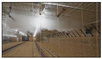
6) Depending on factors such as house width, inlet type, inlet positioning, inside/outside temperature difference, etc. an inlet opening of 2" (+/-1") at a static pressure of 0.10" (+/- 0.02") is generally required to throw cold incoming air near the center of a house.
