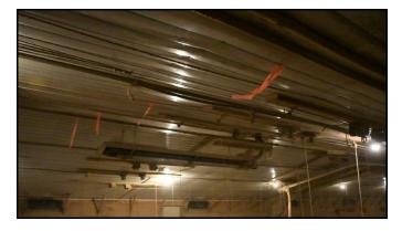
7) 12" pieces of surveying tape should be hung from the ceiling every three to five feet directly in front of an inlet on each side of the house. The goal is to get the surveying tape approximate five feet from the peak of the ceiling to lightly flicker when the minimum ventilation fans are operating.
