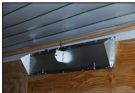
Figure 5. Side "flaps" to prevent air from exiting sides of a galvanized inlet
