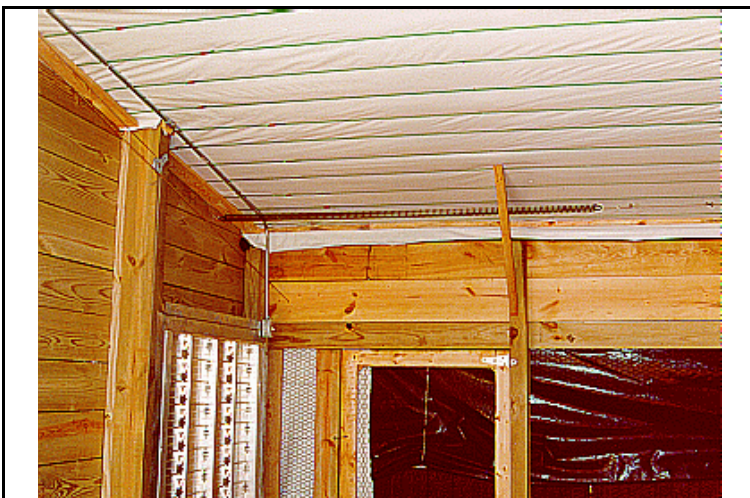
Figure 7. Spring used to pull inlets closed
