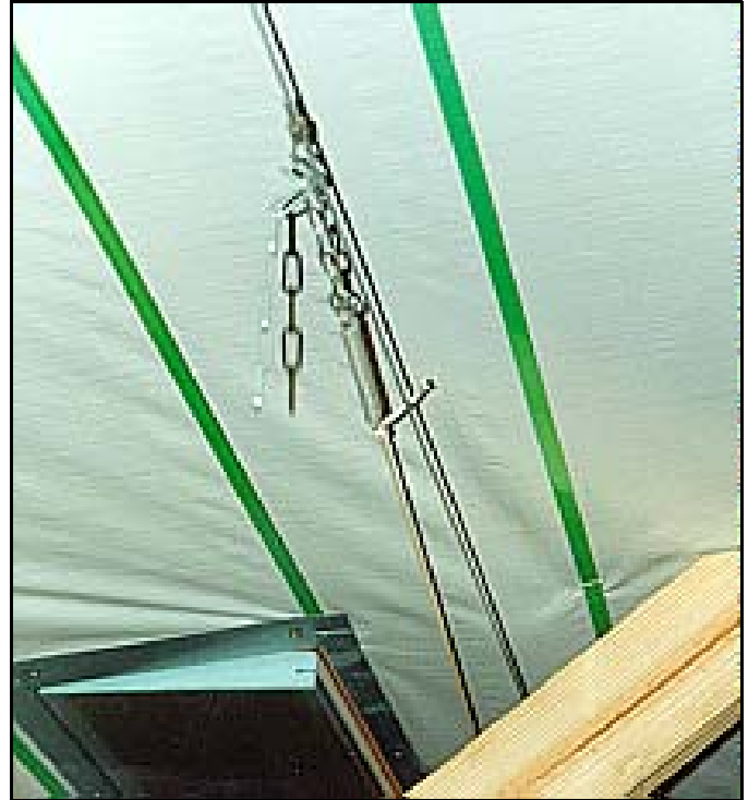
Figure 6b. Small side wall inlet spring and chain.
