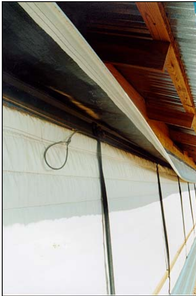
Figure 3. Curtain pocket lifted to view the top of the side wall curtain.
